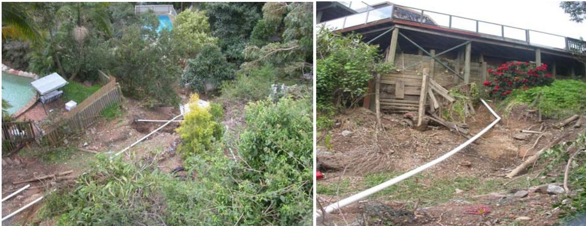
In summary, the claim concerned the failure of a timber retaining wall and associated swimming pool during the heavy rainfall that occurred in the Newcastle area in June 2007.
