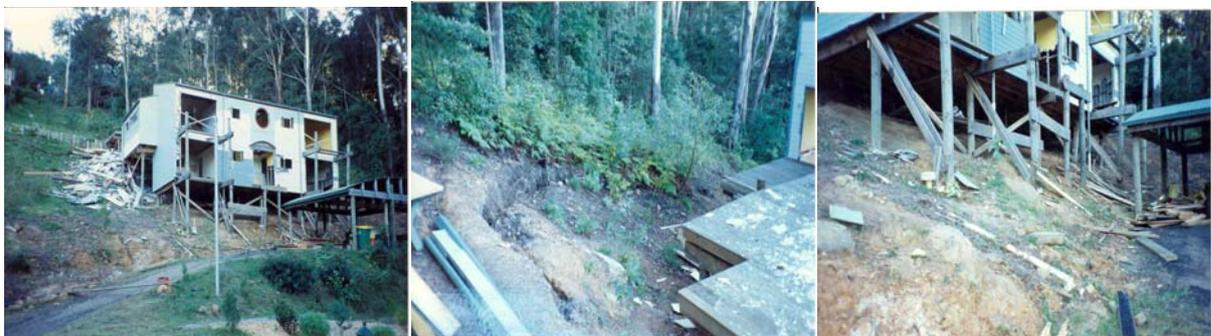
4. When the house was approaching completion, a landslip occurred in the vicinity of, and underneath the house causing the pole footings to crack / break, which then destabilised the house structure and rendered it unsafe.
